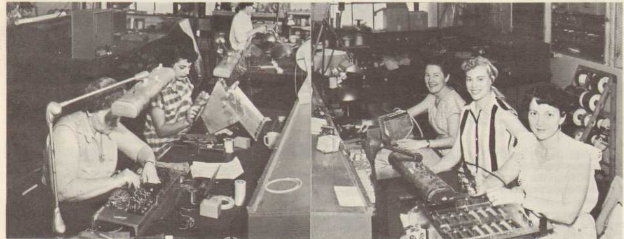
AN LGP-30 IS composed of many parts. Here Lois Miller (left foreground) assembles a power sequence unit while Terry Abbisso wires a logic section. On the right, Epi Bloise solders a memory
