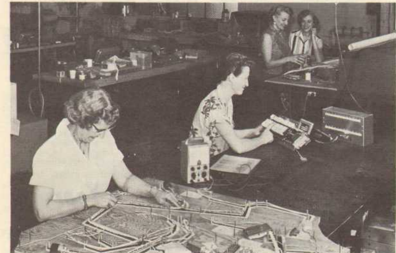
THAT ISN'T A model train layout you see, it's an LGP-30 harness being fabricated by Martha Ries. On her left, Nola Webb checks operation of a control panel. Amelia Burruss and Ruth Gerkin (rear) discuss wiring of a Punched Tape Converter.
