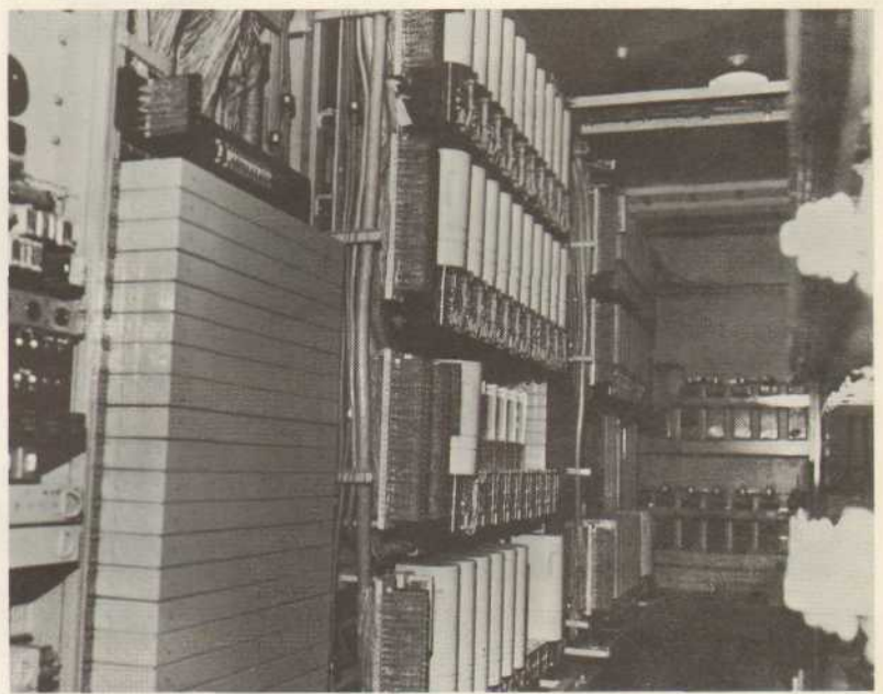
COMMUNICATIONS HUB —This view of Librascope's recently enlarged telephone equipment room in Building 3 gives some idea of the Company's complex phone system—one of the largest private installations in Glendale. The can-like devices in the center of the picture are switching components. In the rear is the battery rack which automatically provides emergency power for the system in case of an electrical failure. (Photo by Duggan)
