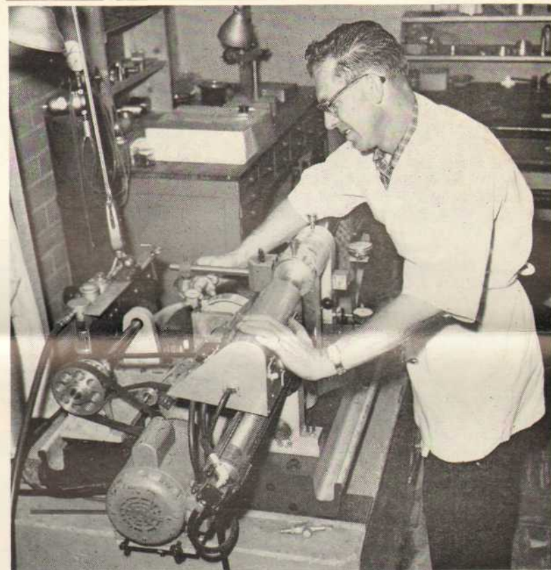
VAN AND MACHINE —Roy W. Van Holm, Prototype Shop Foreman, aligns a CP-209 memory drum on the new precision turning machine he developed. The device, called Van's Drum Machine, is capable of machining drums to tolerances of 0.000050 inch and less. After Van Holm aligns the CP-209 drum to take out its taper, he will check for runout.
