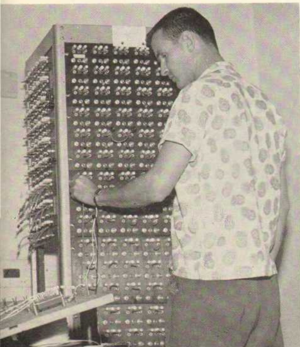
through a transistor for 1,000 hours. At left, technician Joe Parisi is seen preparing a wiring harness which will enable the test panel to have a greater capacity.
