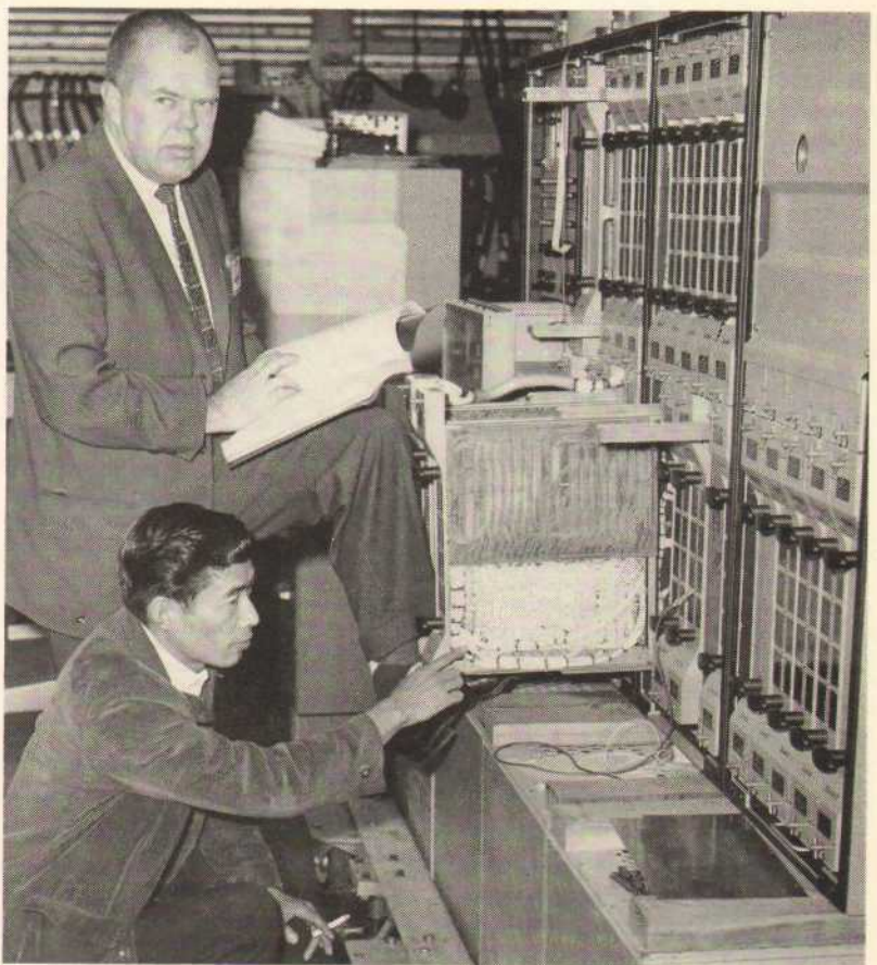
A SIMPLER WAY —Senior Engineer Gray Lange and Designer Peter Iwakami (kneeling) are seen inspecting a portion of the point-to-point wiring on the Micro Program unit for the Mk 130. The wiring on the fire control system was performed with tabulated wire listings, such as the one held by Lange. The new time-saving and cost-cutting method of wiring developed by Lange and Iwakami is the tabulated equivalent of a wiring diagram, accomplished entirely by data processing equipment. The work parallels a similar project undertaken by M. J. O'Neill of the Sunnyvale branch for the FAA data processor.
