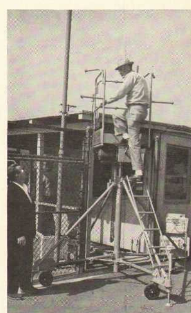
NEW HEIGHTS IN MAINTENANCE —Demonstrating capabilities of the new electric-hydraulic lift recently purchased by Glendale branch for maintenance duty, George Kirby takes a sky-ward trip to change light bulbs. Observing from the ground is Charles Hilgert, Bldg Maintenance Supervisor. A control box on the side of the lift cage allows the man aboard to lower and raise the platform as needed. The caged enclosure and wide platform jacks to steady the lift make it considerably safer than a ladder for the growing amount of maintenance work, Hilgert says.
