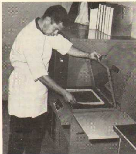
PLATE-MAKER —John Strout readies a negative for the plate-making machine. Impressions are transferred to a metal sheet on which lacquer is applied to produce the printing surface.
