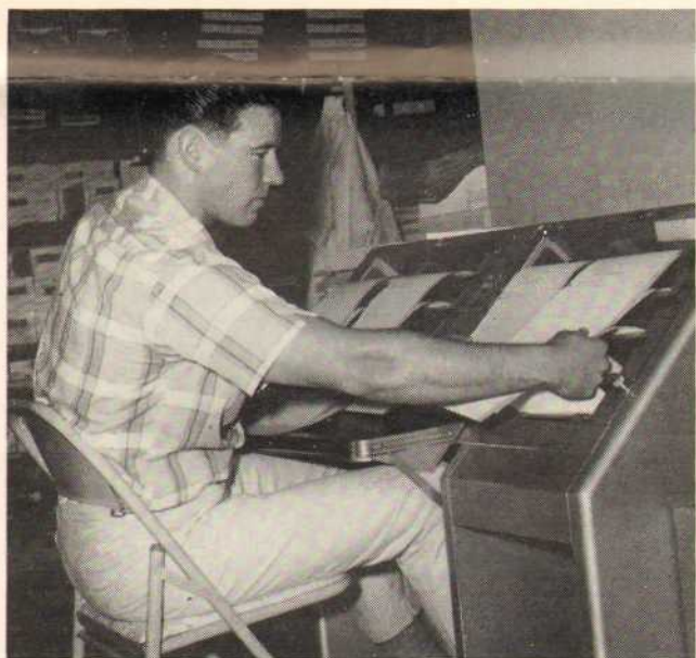
ALL IN ORDER —Gary Buss demonstrates the Collator, a mechanical device which aids in arranging stacks of printed material into proper sequence. With the Collator, the operator can gather as many as 20 pages at one time, all in the right order.
