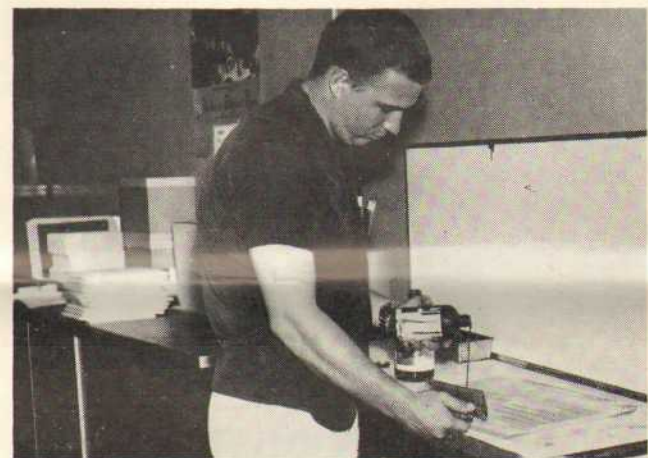
PERMANENT TOUCH —Group Leader Jerry Schweigert finishes a permanent master sheet for the offset process by adding lacquer to form the printing surface on a metal base. Metal master sheets permit a multitude of reprintings without loss of clarity, and they can be easily stored for future use.
