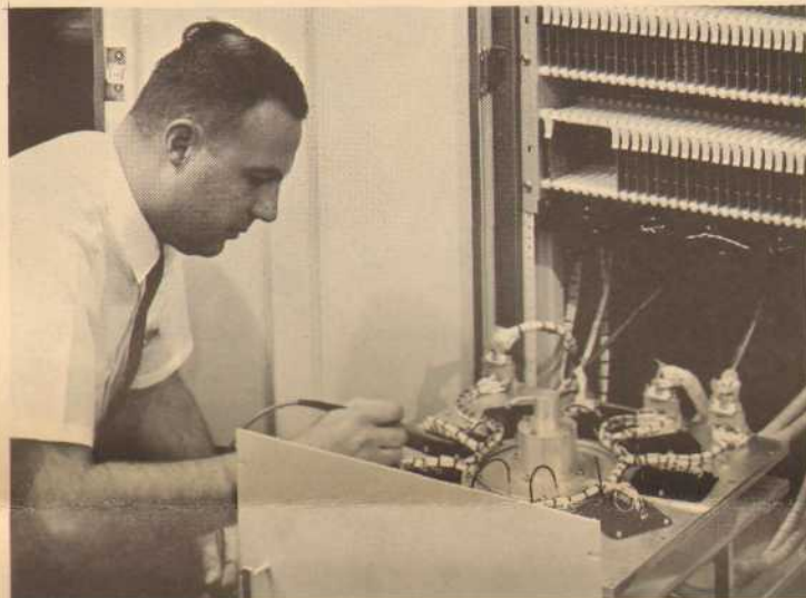
PARIS AIR SHOW—Jim Rosdorff, Components Division Engineering, checks read/write heads on a Librascope L416 disc memory. The L416, along with a new Hybrid Encoder, are among Librascope products to be exhibited at the Paris Air Show this year.
