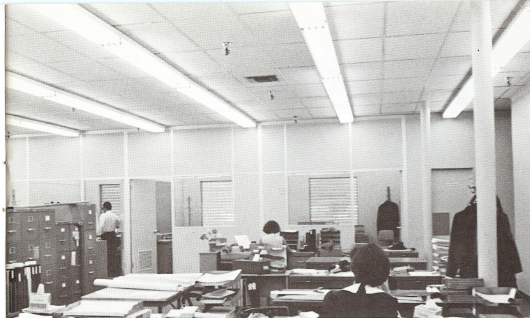
Improvements in Engineering, Bldg. 1, include expansive use of glass on perimeter office walls, acoustic ceilings and improved lighting.
