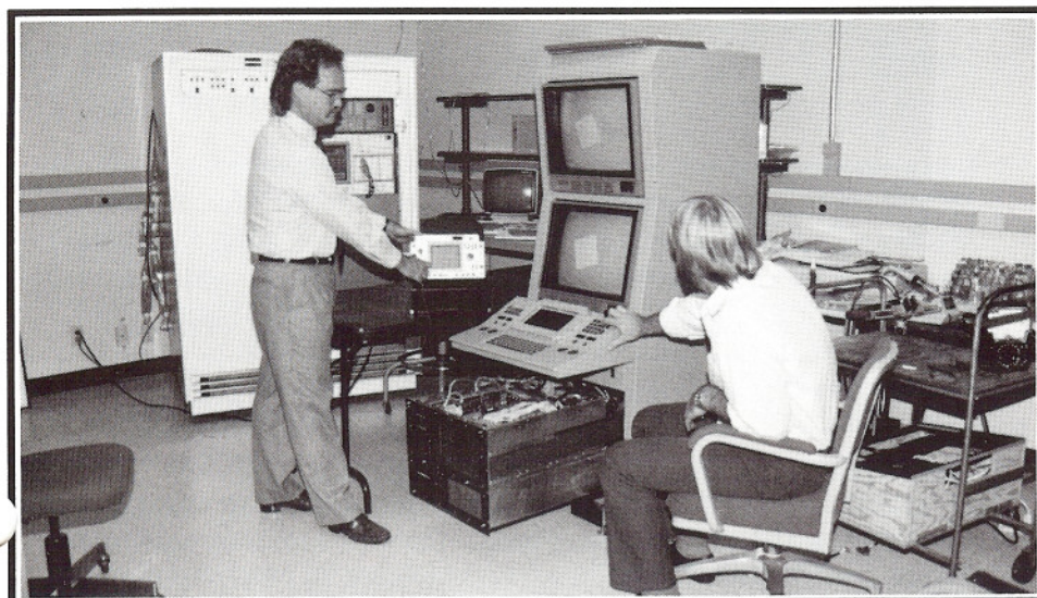
Ed Wanek, left, Supervisor, Test Equipment Design, explains the operation of the Combat System Display Console (CSDC) Automatic Test Equipment (ATE) to Joe Killian, Sr. Electronic Technician.
