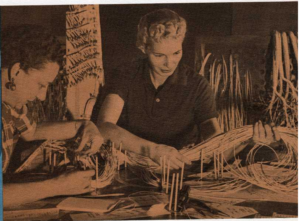
Great skill and experience is required to assemble the main harness which comprises the "nerve" system of a Librascope Analog Computer.
