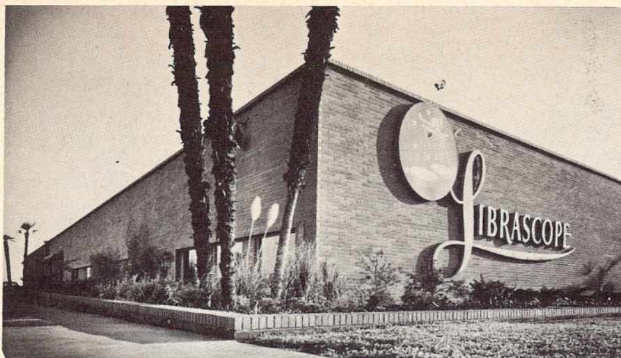
Administration and engineering headquarters of Librascope in Glendale.
